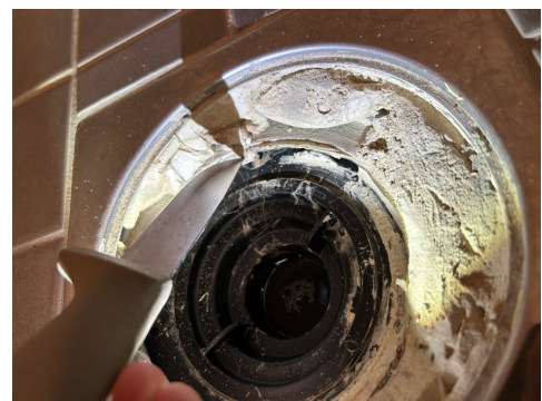
Plastsluk, membran under klemring.
