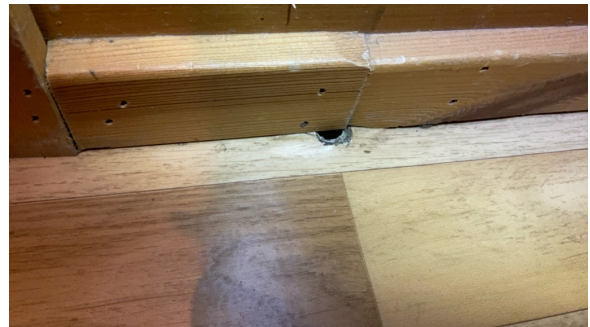
Hull i belegg
